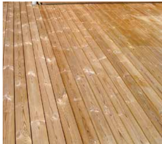
4. The deck was yellowish brown at first, because the wood protection is alkaline. The silicon-based wood protection then began to have in-depth effect to protect against pests and to strengthen the wood. A clean and light wood surface emerges over time.
