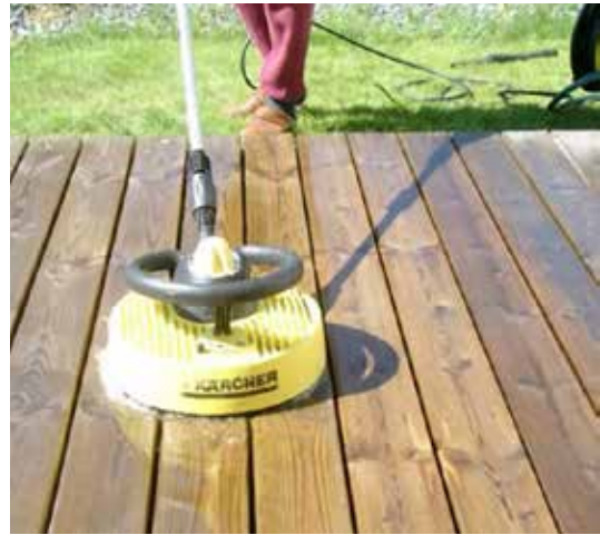
2. ...with alkaline cleaner, brush and rotating pressure washer.
