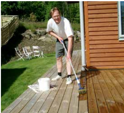
3. When the deck was dry they applied two coats of Premium Wood Protection Deck. When this had dried, after about four hours, they then applied Premium Surface Protection Deck.
