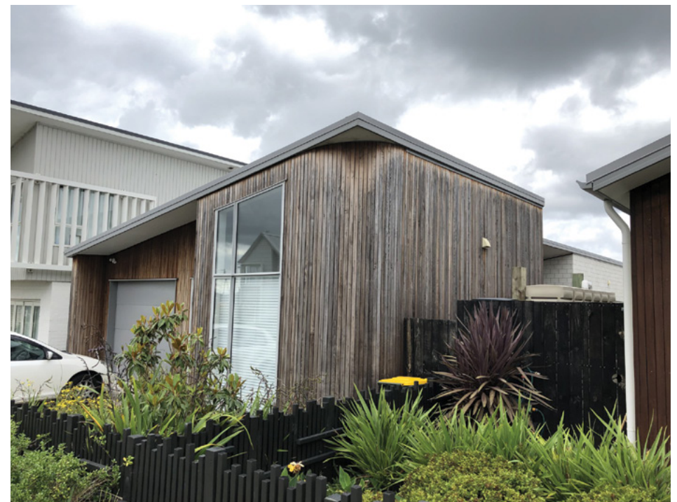
○ Uneven weathering of uncoated Western Red Cedar.
