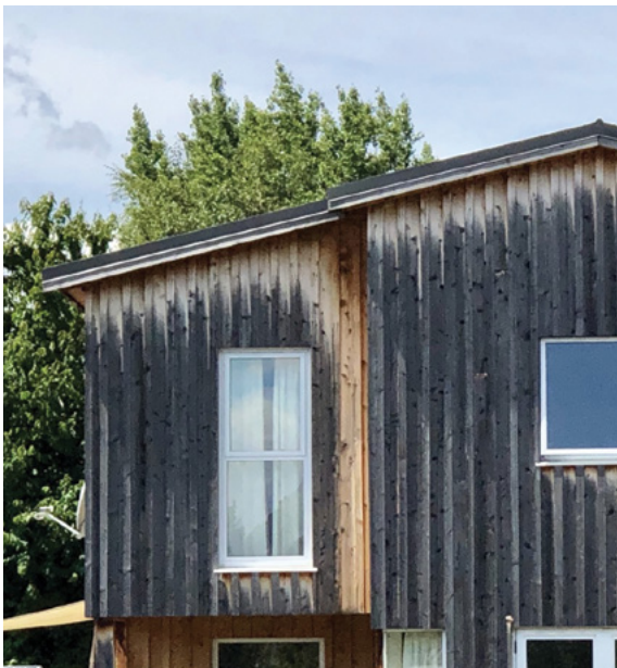
○ Surface mold (black mold) – Larch.
