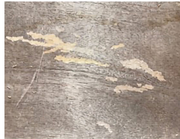
○ Paper Wasp damage.
