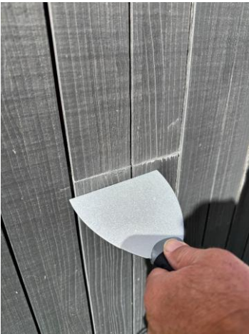
Ohinewai site office – Scarf joins
