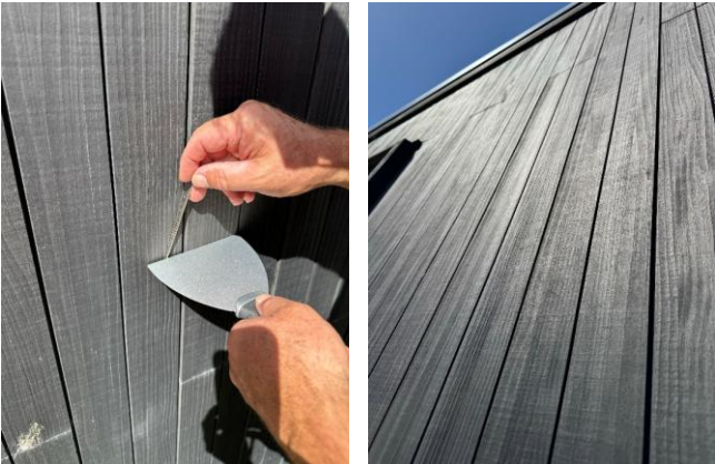
Ohinewai site office – Cladding minimal dimensional movement, no checking
