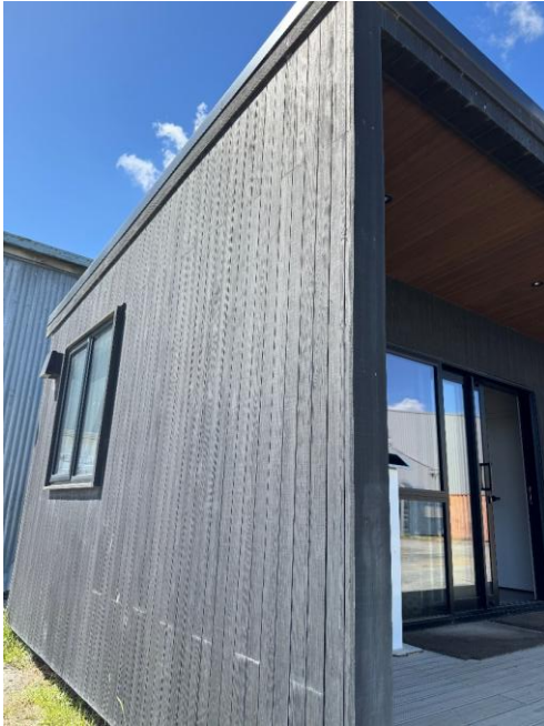
Ohinewai site office – Vulcan Engineered WB12 138x20 Nero, north wall.
