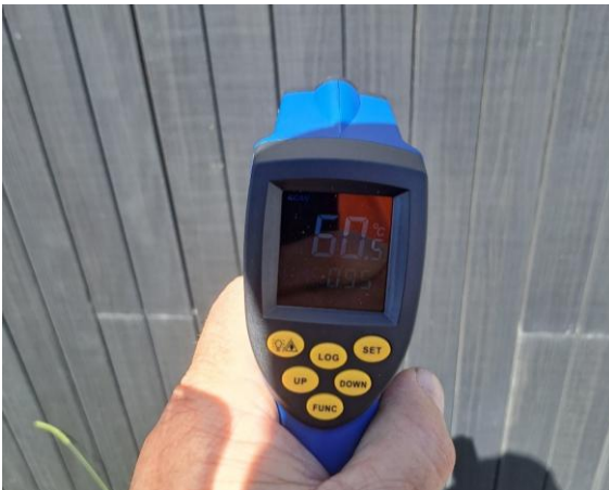
Ohinewai site office – North elevation summer temperature 1pm
